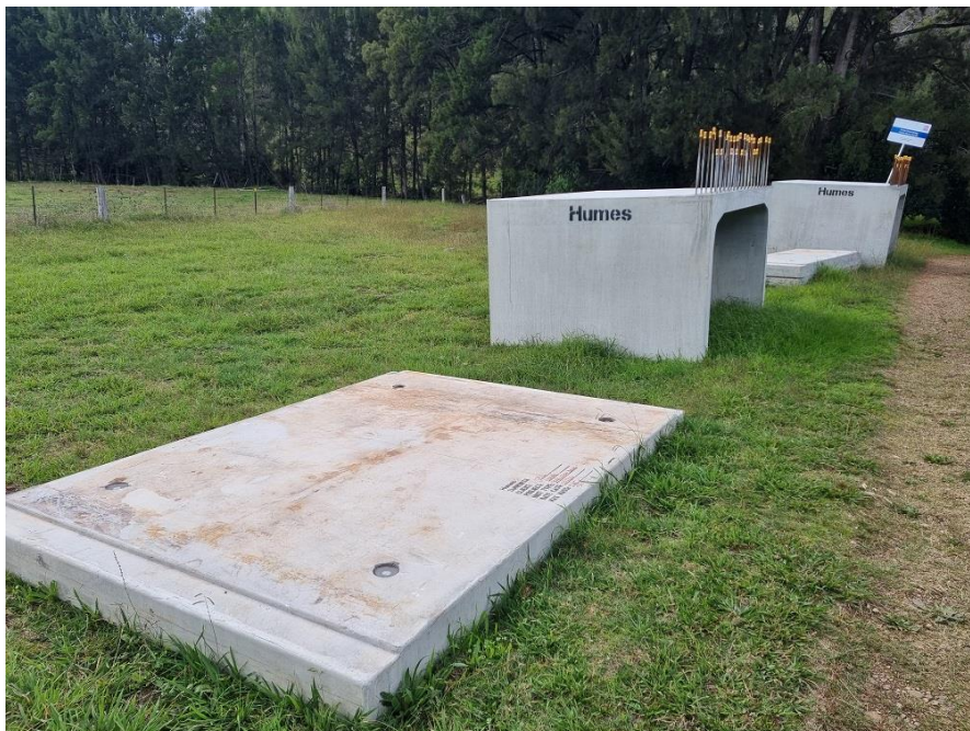
Figure 3 – Culvert precast components on site
